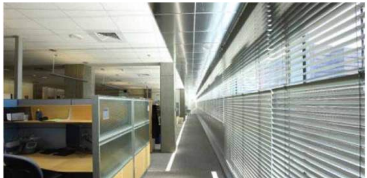
FIGURE 4.5.1 | USE OF HORIZONTAL BLINDS IN OFFICES (TAKE NOTE OF THE BRIGHTER CEILING AND REFLECTIVE CEILING USED IN THIS PICTURE)
