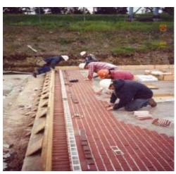
Figure 1: Laying the thin bricks
