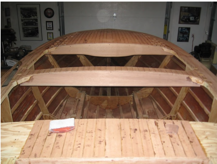
“Mahogany deck surface being installed.”
