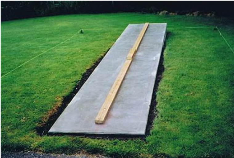
“The concrete slab to build the jig on.”
