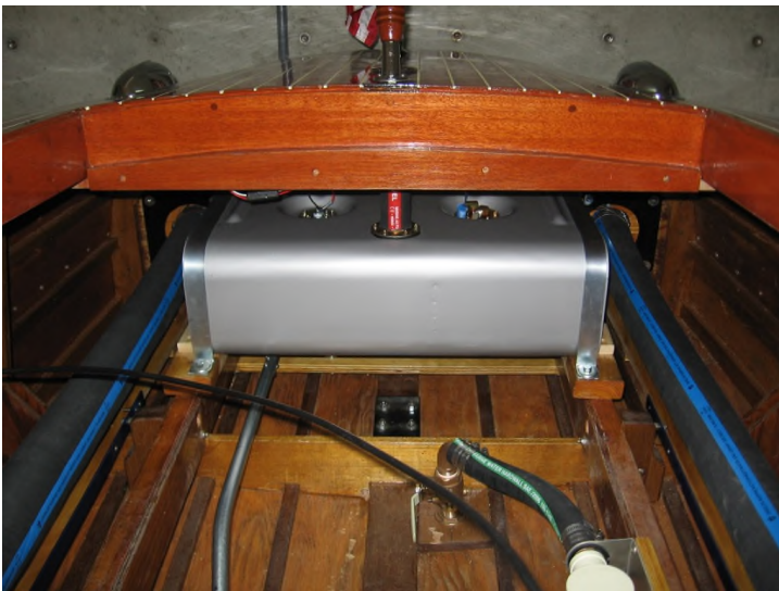
“Fuel tank installed. Exhaust tubing installed and connected to exhaust ports.”
