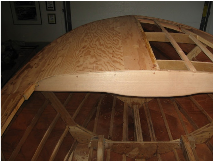
“Sub deck sheathing being installed.”
