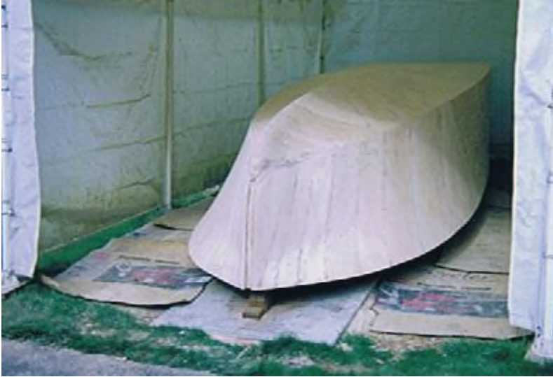
“The hull sub-sheathing is complete and ready for installation of mahogany sheathing.”
