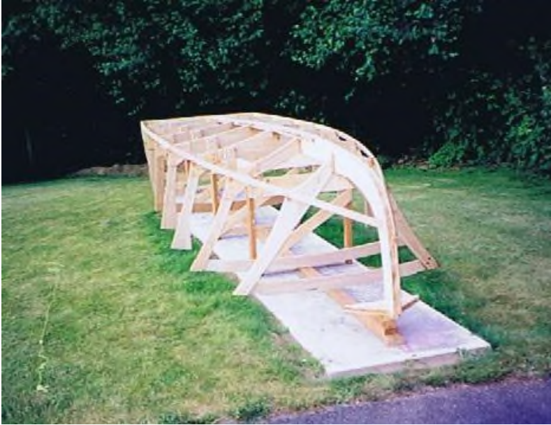
“The framing on Jig beginning to take shape.”
