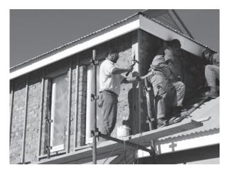
Supporting timber structure used on masonry walls should not be less than  $38 \text{ mm} \times 38 \text{ mm}$ .
