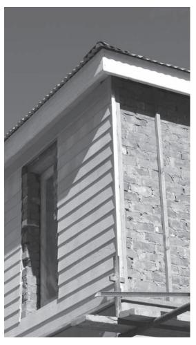
The distance between vertical supporting timber or metal studs should not exceed 600 mm.
