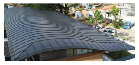
[Figure 17] Flexible amorphous silicon laminates glued to a curved metal roof (Sentosa Cove). Photo courtesy of Sheet Metal International
