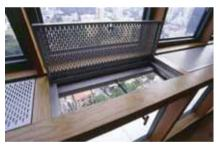
[Figure 21] Monsoon windows allow wind movement into the unit without allowing rain to penetrate into the unit. Photo courtesy of Tim Griffith Sketch © WOHA All Rights Reserved
