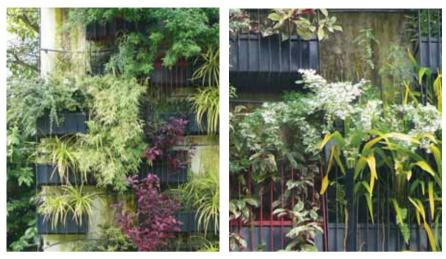
[Figure 11] The plant-cassette system (left) and its close up (right).
