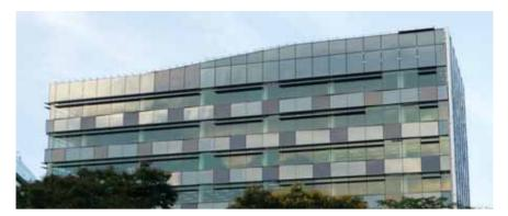
[Figure 14] Amorphous silicon BIPV modules (dark squares) integrated into a façade (No. 7 Tampines Grande). Photo courtesy of Phoenix Solar
