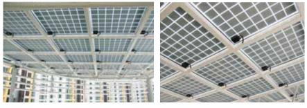
[Figure 15] Crystalline silicon BIPV modules integrated into a skylight canopy (Savannah Condo).
