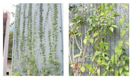
[Figure 9] The modular trellis panel system (left) and its close up (right).
