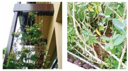
[Figure 10] The cable and wire-rope net system (left) and its close up (right).
