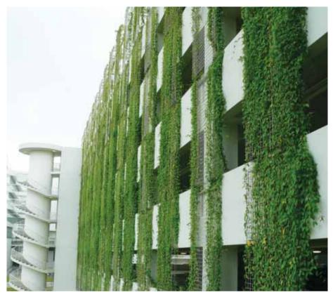
[Figure 15] The green façade of the multi-storey car park at Republic Polytechnic.
