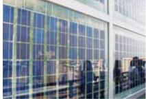
[Figure 16] Crystalline silicon BIPV modules integrated into a façade (Biopolis).
