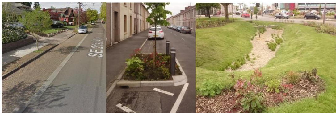
Figure 16: Examples of blue-green interventions: Left: Street permeable paving edges. Centre: Street planters. Right: Detention basins/
