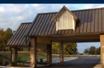
Weather Lok-16 is a mechanically seamed roof panel. It is available in 24 gauge only.
