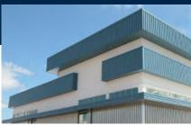
7.2N Rib can be used for wall and roof applications. It is available in 29, 26, 24, and 22 gauge.
