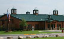
Super Seam II is a snap sealed standing seam roof panel. It is available in 24 gauge only.
