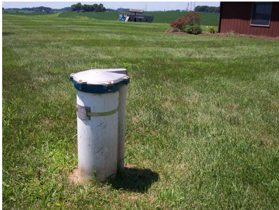
Figure 4- Completed Well with Casing, Tag, Cap, and Conduit
