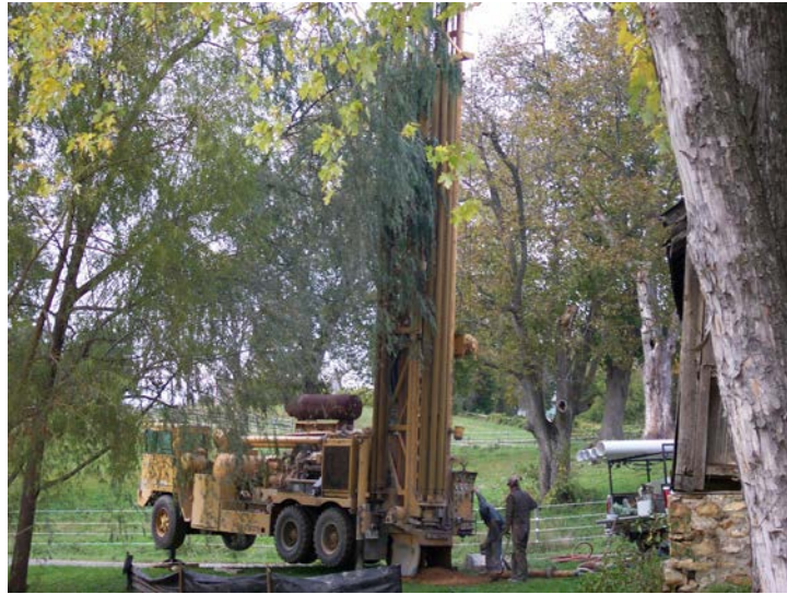
Figure 3- Well Drilling Rig
