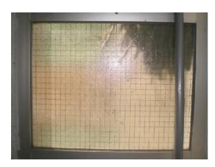
There are a number of things which can be done to a window, in order to make it stronger and better to withstand attacks. The first of these is to replace all the window glass with the wire glass that is used in industrial facilities. While this isn't a perfect solution, it is much stronger than normal glass.
