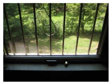
Burglar bars are wrought iron bars which form a grating over the window. They are anchored into the brick or studs on the outside of the home. Once anchored, it is typical to grind the bolt heads, so that they cannot be removed.
