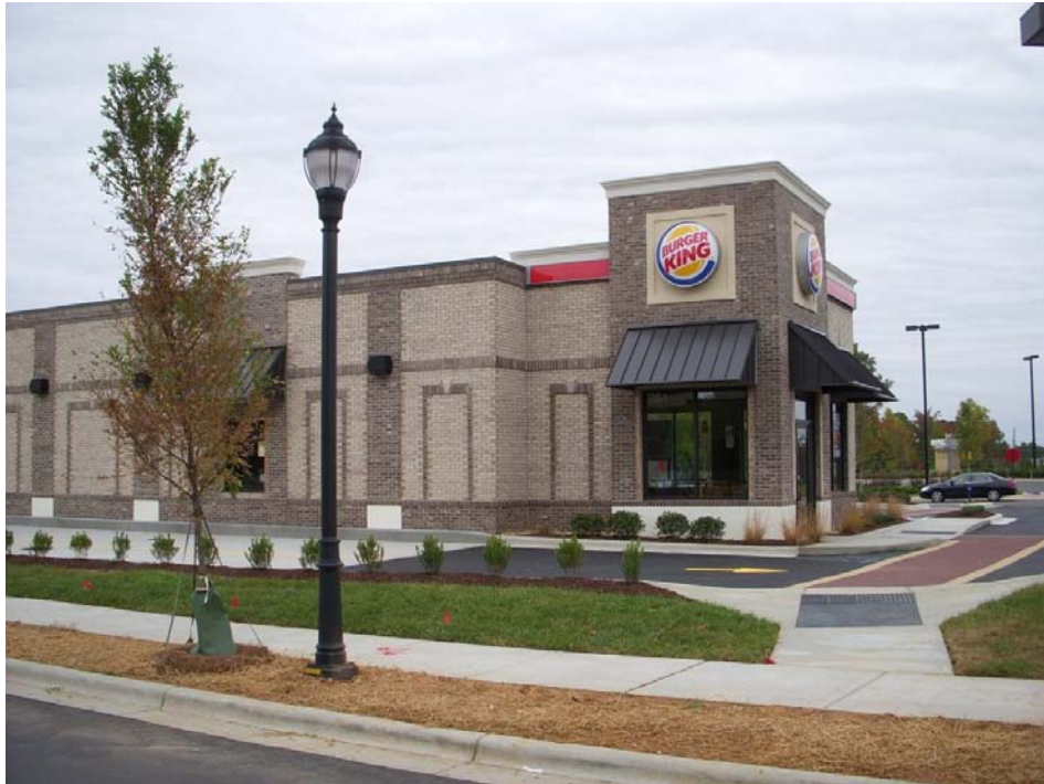
Photograph 3.04 – ACCESSIBLE PATH OF TRAVEL FROM RIGHT-OF-WAY
