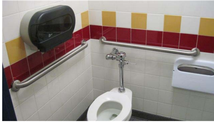
Photograph 12.09 – TYPICAL RESTROOM PHOTO
