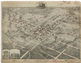
First sewer lines were constructed around the Courthouse in the early 1900s
