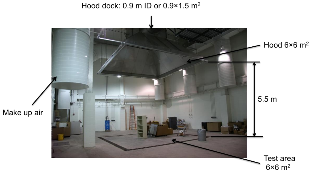
Fig. 30: WPI-facility for large-scale test
