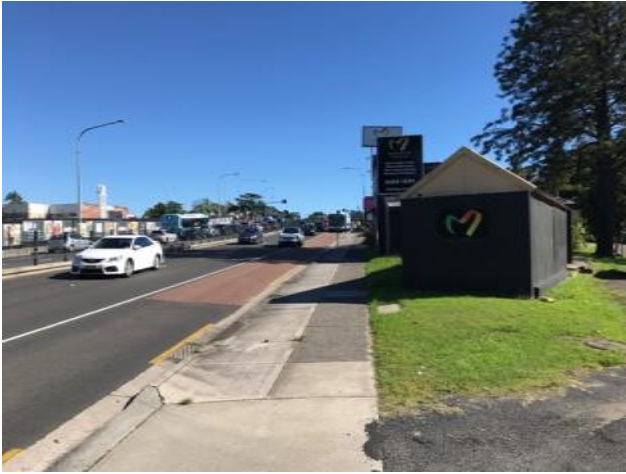
#28 View north towards existing stop 2153226 with new location in foreground
