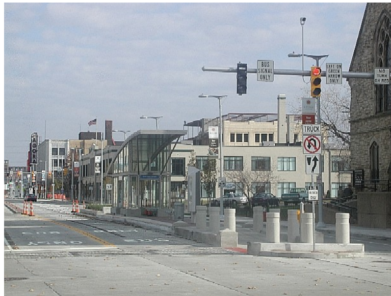
Median station with side platform for right-side boarding (Cleveland HealthLine).
