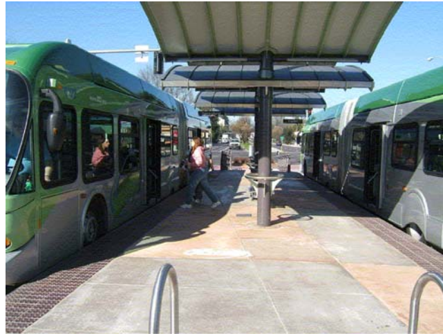
Median station with center platform (Eugene EmX).
