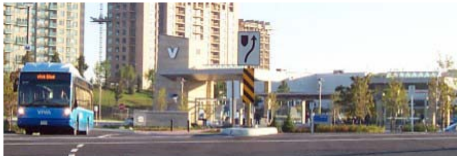
VIVA Richmond Hill Transit Center (York Line).
