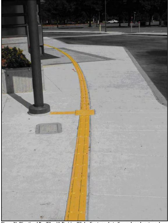
Figure 31: Directional Bar Tile with Decision Tile leading to an electrolier used as a bus stop pole. Location: West Valley College, Saratoga.
