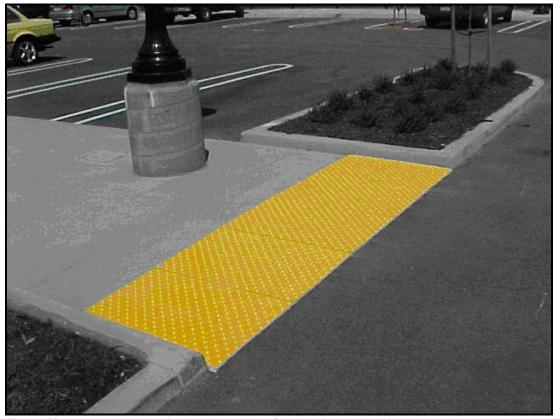
Figure 38: Detectable Warning Band at edge of pedestrian path adjacent to vehicular roadway Location: Mountain View Transit Center
