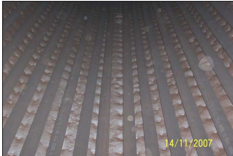
Figure 4. Internal visual inspection of radiant coil tubes
