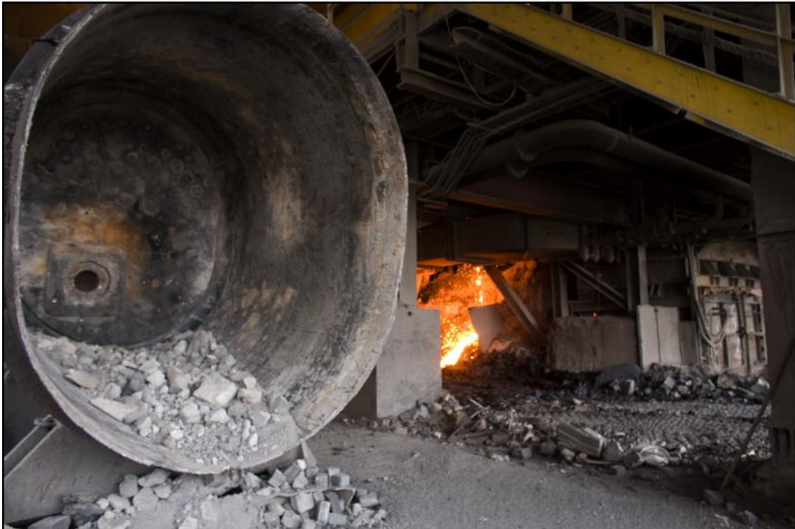
Knowing the exact amount of scrap metal placed in the furnace allows Nucor to precisely calculate the amount of electricity required to heat the furnace.
