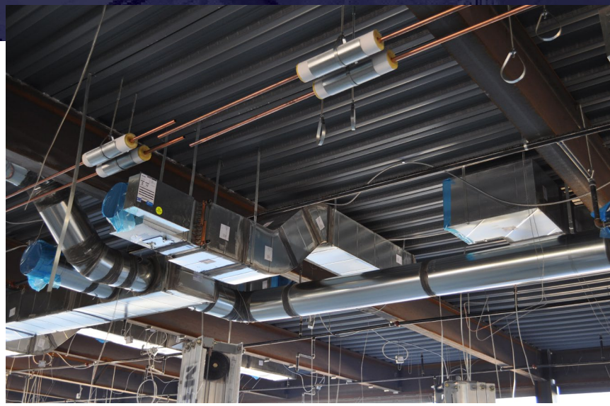
MEP coordination using BIM technology in advance of field installation eliminated fit issues.
