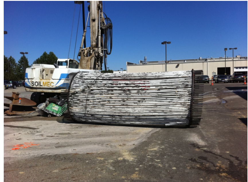
Photo from Byers and Renier Construction, NREL/PIX 18814
