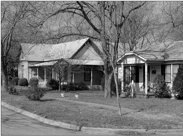
In residential areas, most roof forms are pitched, such as gabled and hipped.
