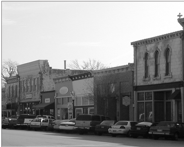
Most commercial buildings have flat, or slightly sloping roofs.
