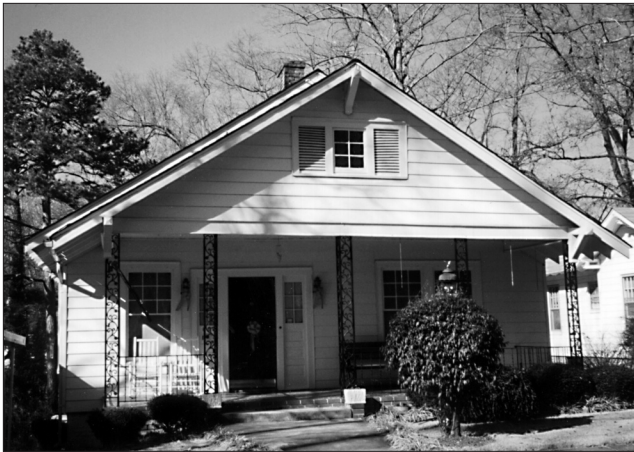
This porch has experienced an inappropriate alteration; wrought iron supports have replaced wood piers. Compare it with its “twin” in the photo below. (Spartanburg, SC)
