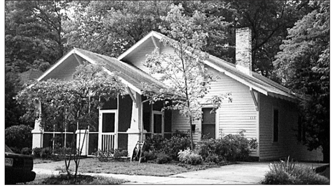
When a porch is enclosed or screened, it shall be done with a clear transparent material. This material should be placed behind porch columns. (Memphis, TN)
