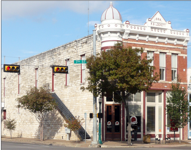
The side wall of a historic building located on a corner will have fewer openings.
