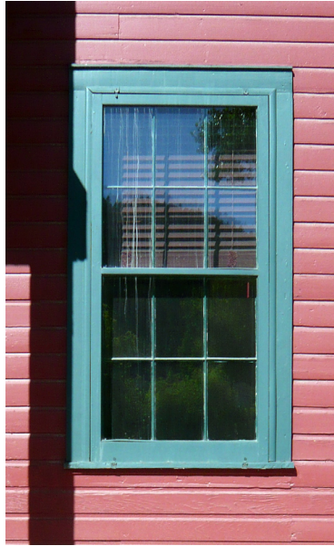
Consider use of a storm window to enhance the energy efficiency of an existing historic window rather than replacement. (Deadwood, SD)
