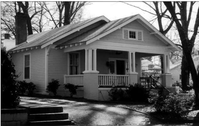
When replacing porch posts, use supports that are of adequate size. This porch reconstruction was based on neighboring houses of similar character and age. (Spartanburg, SC)
