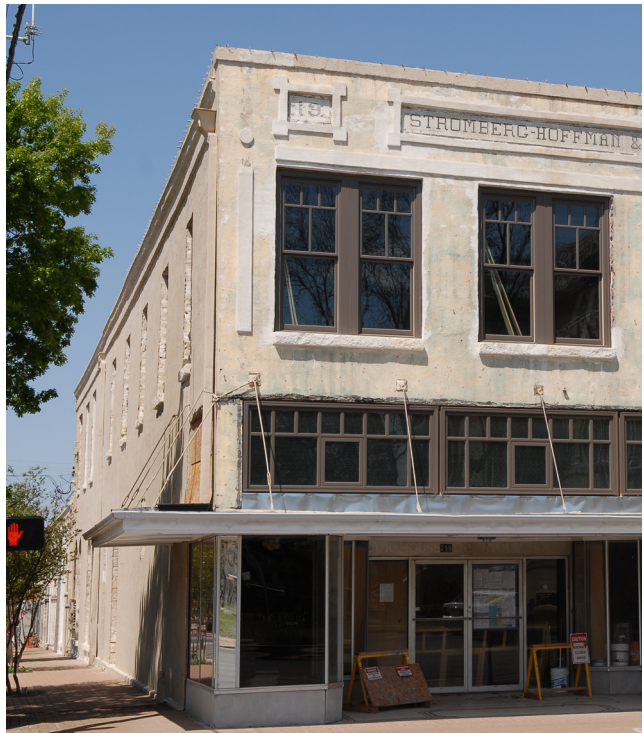
After: The upper-story windows have been reopened.
