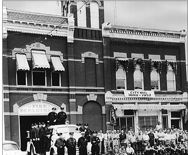
Using historic photographs can help in determining the original character. (Compare with below.)
