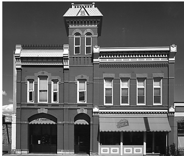
This rehabilitation preserves surviving details and reconstructs missing ones. (Ft. Collins, CO)
