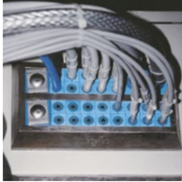
Captain's bridge: Route wiring through Roxtec cabinet seals and into enclosures without compromising IP ratings.
