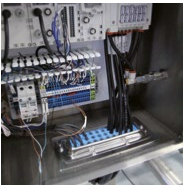
High pressure wash down environments: The Roxtec CF 16 AISI 304 maintains high sanitary requirements.
