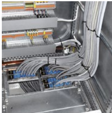
Control cabinets: The Roxtec CF 32 PE for potential equalization is used for generator and turbine cubicle marshalling.
