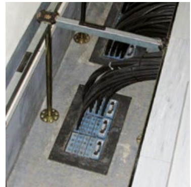
Communication centers: The Roxtec GHM solution seals fiber optics and cables in floors and outer walls.
