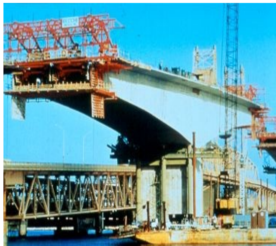
Figure 1.9 - Cast-In-Place Segmental construction using Form Travelers
