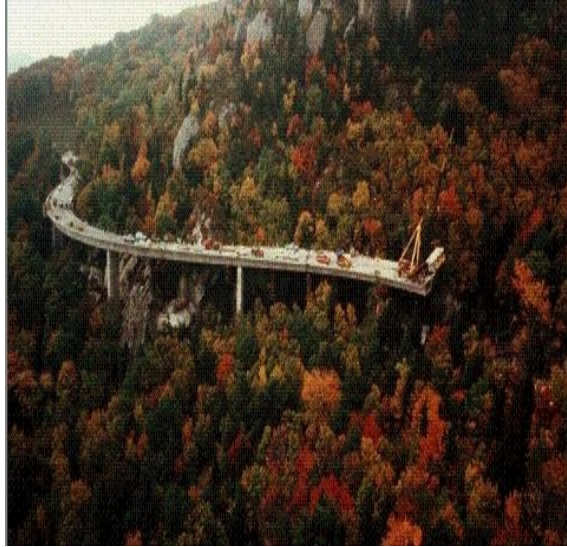
Figure C.9 - Construction of the Linn Cove Viaduct
