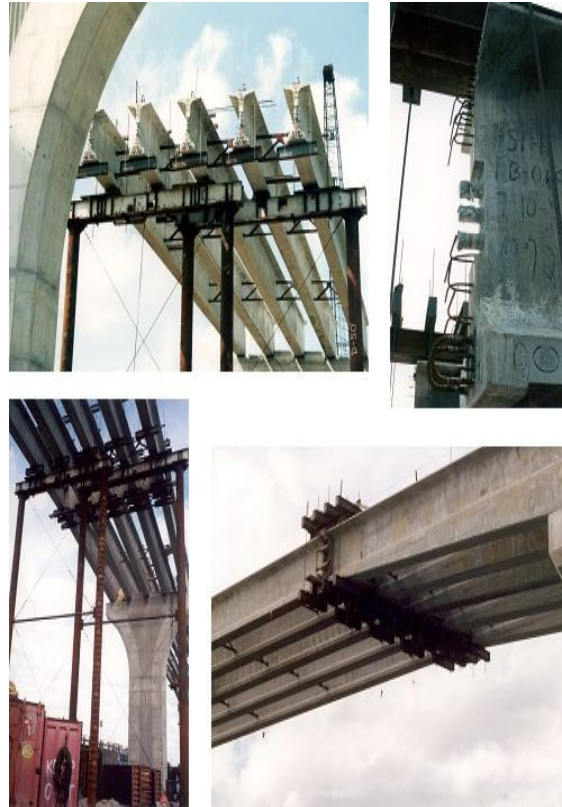
Figure 1.7-Spliced Haunched I-Girder of Main
