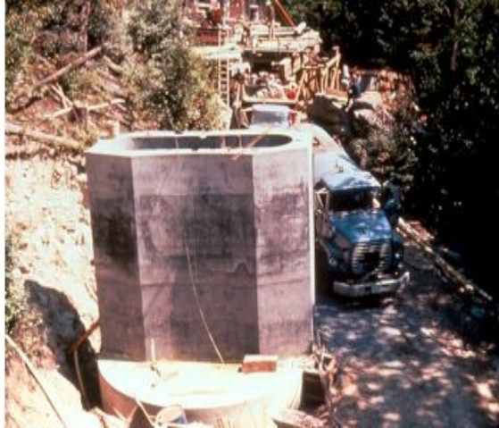
Figure 1.19 - Precast Hollow Segmental Piers, Linn Cove Viaduct, North Carolina
