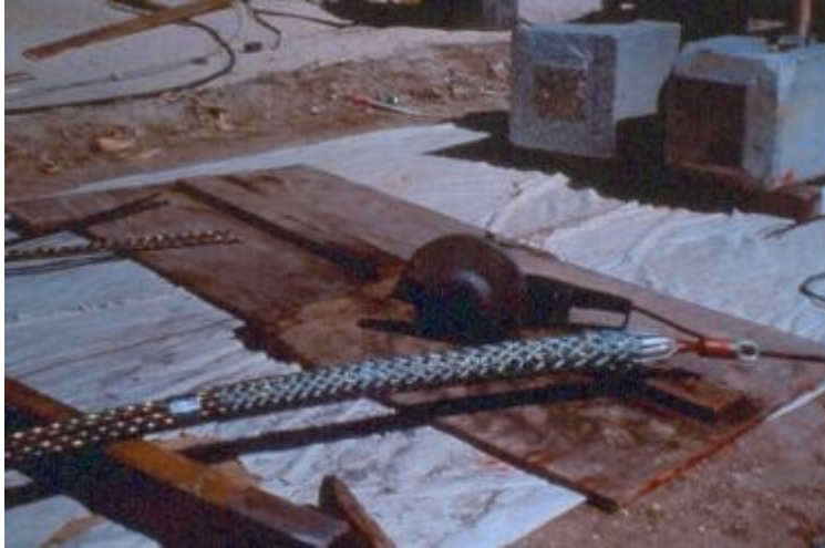
Figure 3.25 - Steel wire sock for installing multi-strand tendon
