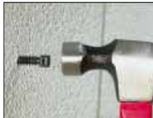
2. Hammer mount into hole.
