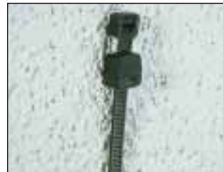
3. Place cable tie through mount.
