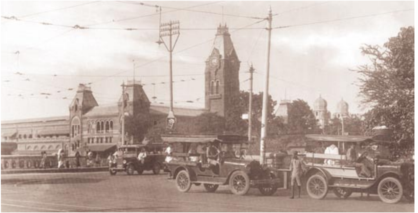
The headquarters of The Madras and Southern Mahratta Railway, predecessor of the Southern Railway.
