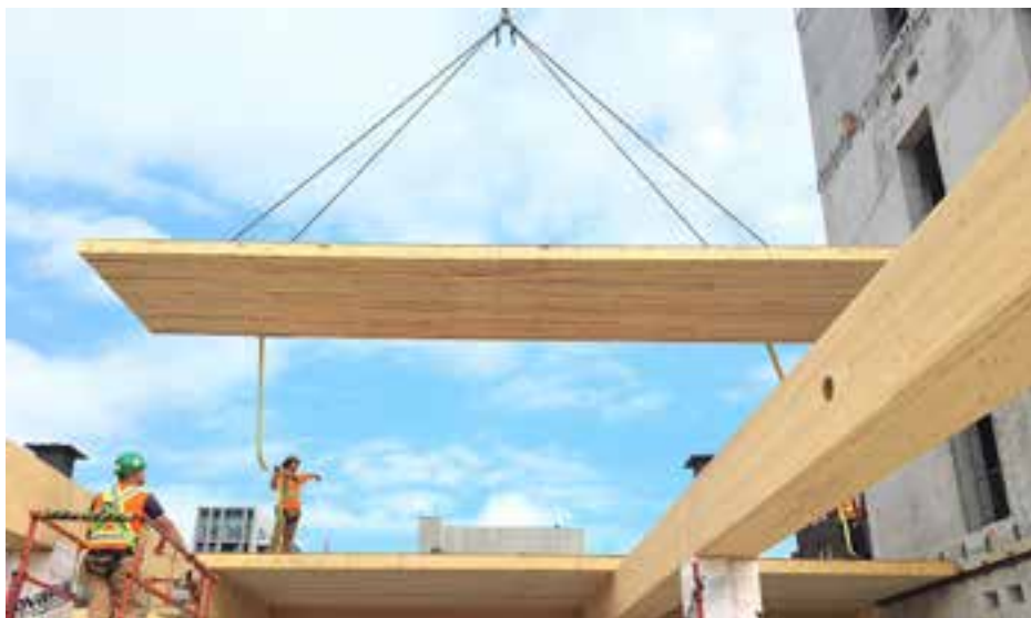
Raising Crew lifts NLT panel into place.
