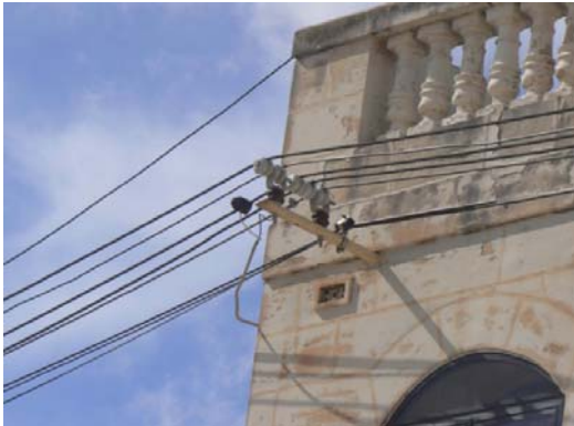
Figure 3.6: Part of the electricity infrastructure – Melita’s cable is the heavy black one [Source: Analysys Mason, 2012]
