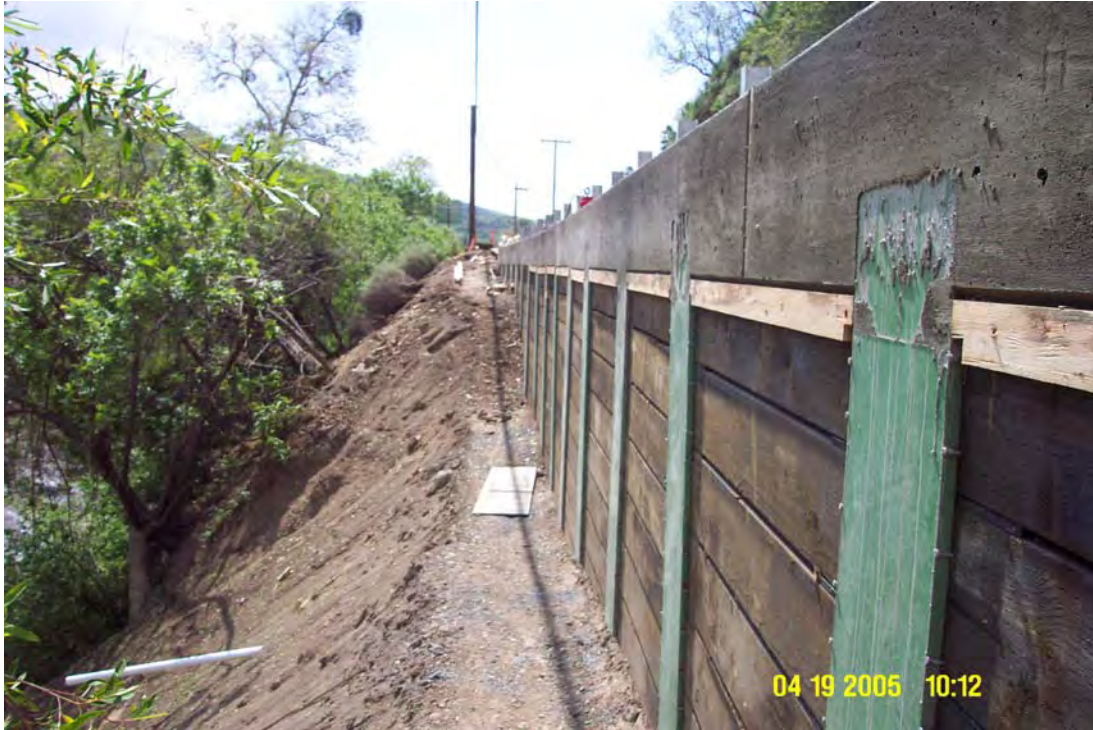
Figure 6-2. Soldier Pile Wall with Cap Beam
