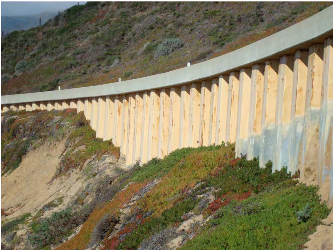
Figure 6-1. Sheet Pile Wall with Cap Beam
