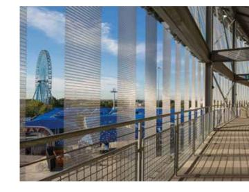
We used two different scales of mesh, which became a design tool. We placed long ribbons of smaller scale stainless mesh from the top of the structure all the way down to the bottom. Then, on the upper portion of the structure, we used the larger scale stainless mesh that reflects much more sunlight. When we overlap the two, you sense the depth between both patterns as it transforms the surface into a diaphanous veil.
