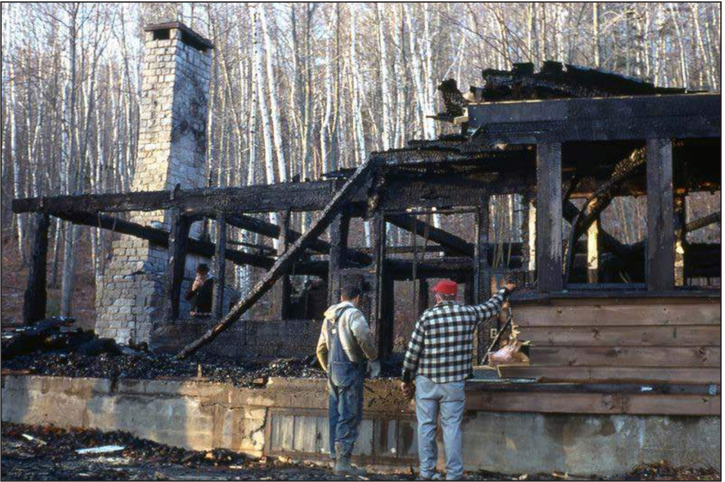
The original base lodge at the Camden Snow Bowl burned in 1967. Above, Sonny Goodwin (left) and Snow Bowl general manager Ken Hardy examine the ruins. Goodwin's construction company, Monroe and Goodwin, would build its replacement. (Courtesy Sonny Goodwin)
