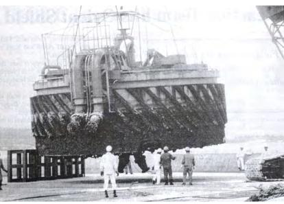
A defective 150 ton monobuoy is removed by members of the 505th Quartermaster Battalion on Okinawa to be replaced by a refurbished one in 1999. The 10 meter buoy is used for unload fuel from tankers.
