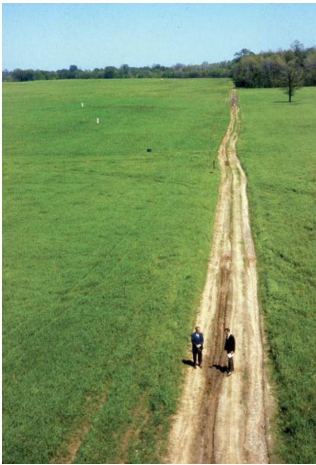
Above, in 1964 RIT President Mark Ellingson surveys the 1,300-acre field that would become the modern RIT campus in Henrietta. At right, work on the main entrance begins later that year.
