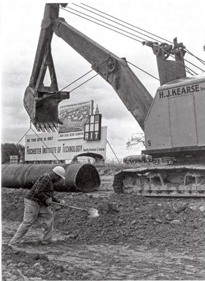
Installing culvert under main entrance road - 8/12/64
