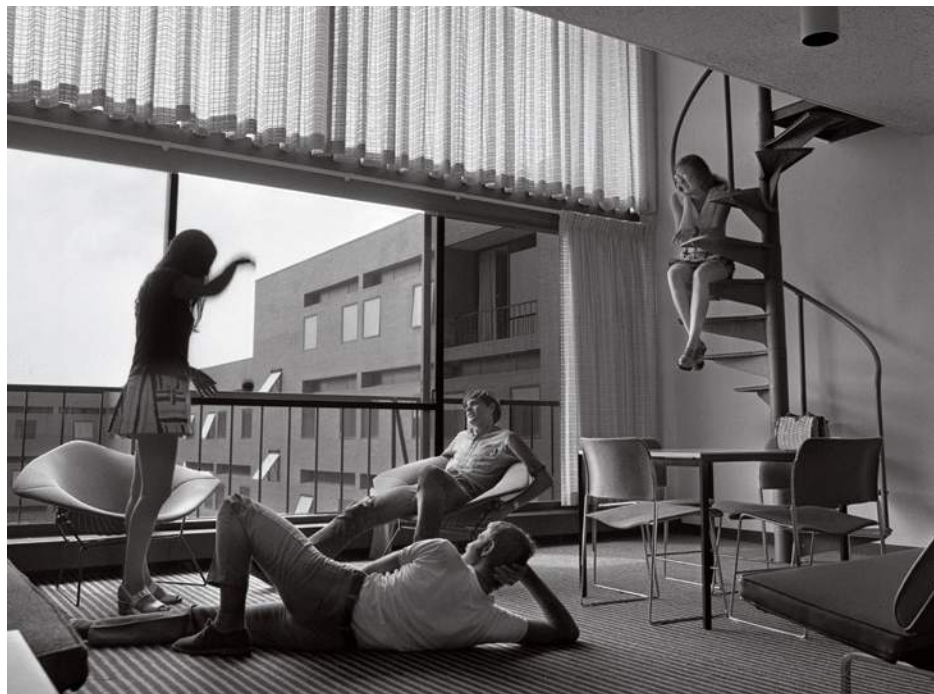
Students relax in a lounge at the new Henrietta campus in 1970. The two-story common areas were renovated to single-floor rooms in the ‘90s to create more useable space in the residence halls.
