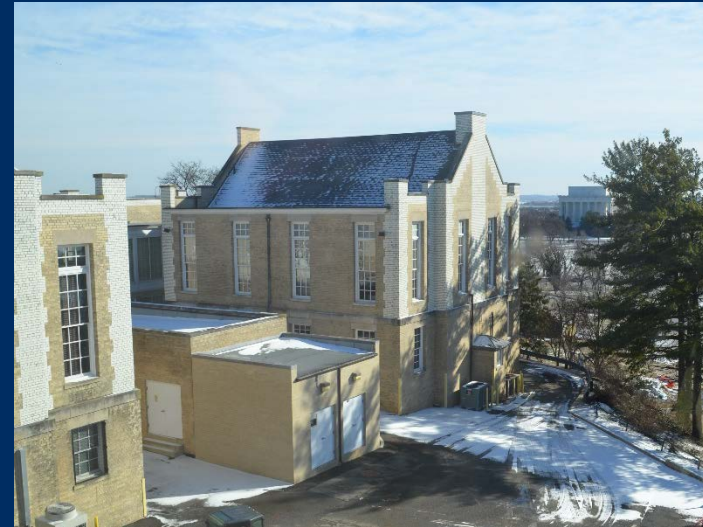
Southwest Ward, North Elevation
