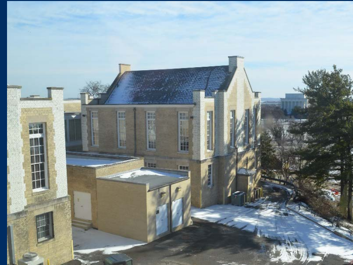
Southwest Ward, North Elevation
