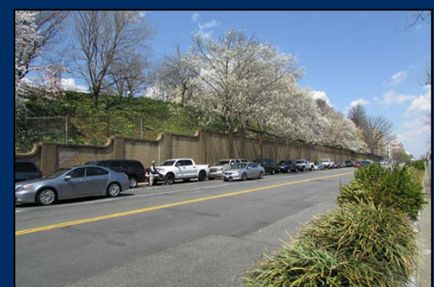
23 rd Street Retaining Wall
