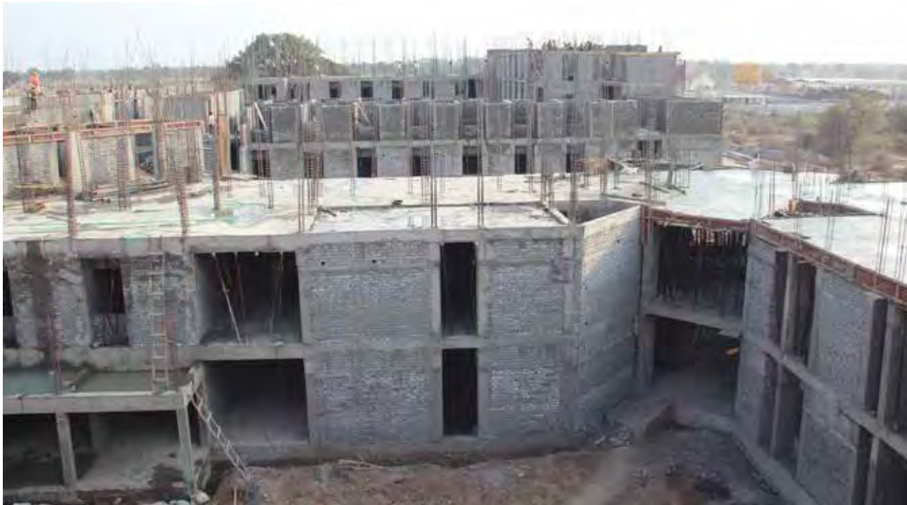
Hostel buildings under construction
