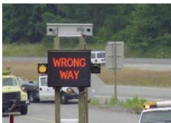
Figure 5.6.16–5: Example of LED-Enhanced Wrong-Way Signage
