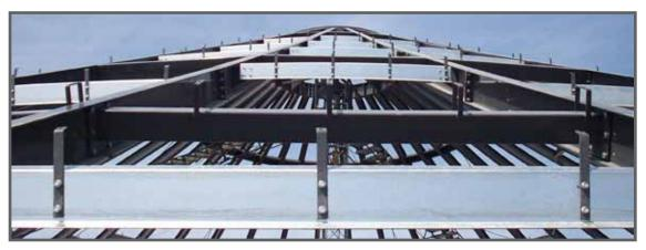
The roof panels are attached to the roof skeleton with standing seam roof straps (above) minimizing penetrations in the valley and creating a more weather tight roof. The roof panels are rigidized (right) across the entire width to produce a more rigid panel for longer life. The roof panels attach with numerous bolts to the wall system through a continuous angle (below) at the eave. This Behlen feature prevents roof panels from tearing loose in high wind conditions.
