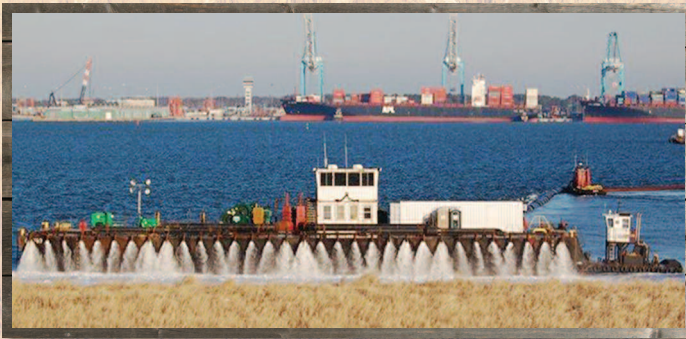
Spill barge building the foundation for the Craney Island Eastward Expansion.
