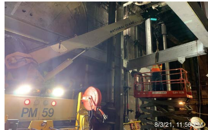
Construction of fan platform in tunnel shaft
