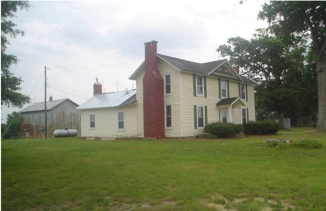
Overall view of house and barn
