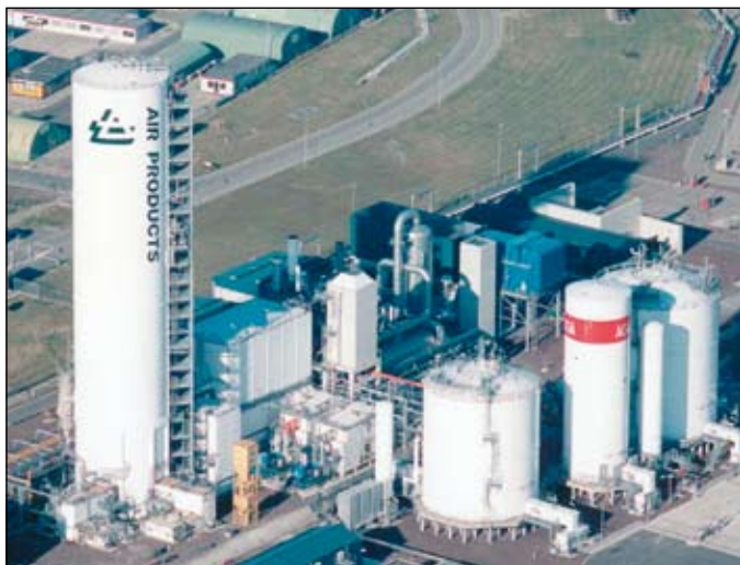
Figure 3.12b A 3000 t day -1 oxygen plant (Courtesy of Air Products).
