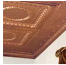
FILLER PANEL AND CORNICE APPLICATION
