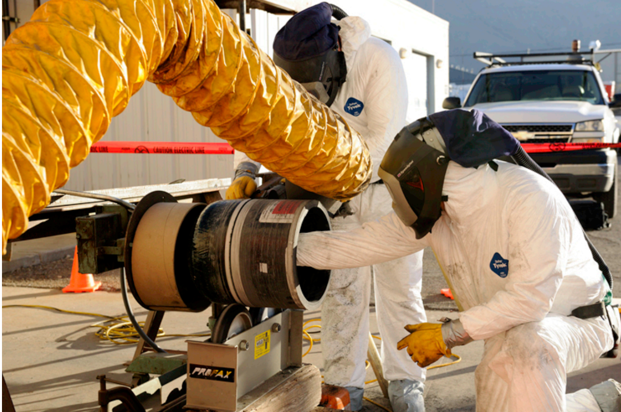
Figure 17 Cutting Operation with Dust/Fly Collection, Ventilation, and Filtration System
