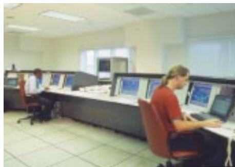
The control room building was completed in 1999 to house a computerised Integrated Control System [ICS]. When operational, this system will automatically monitor our plant and T&D system while providing operators with more accurate and timely information.
