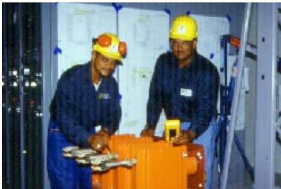
Derron Watson, Industrial Electrician Apprentice, and James Sherieff, Industrial Electrician, of the Electrical Maintenance Department.
