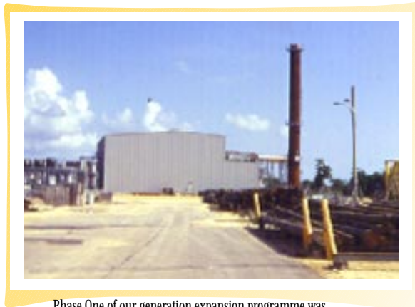
Phase One of our generation expansion programme was completed in the summer of 2000 with the construction of a new engine room, which houses two MAN B&W 12.25 MW V48/60 units along with a 140-foot exhaust stack. This US$30 million project is part of our 10-year strategic alliance agreement with MAN B&W Diesel AG of Germany.
