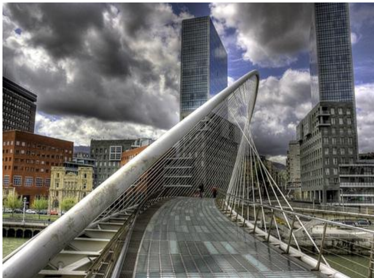
Figure 6: Zubizuri Bridge in Bilbao Spain
