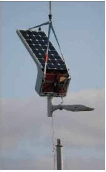
Hoist unit into place
