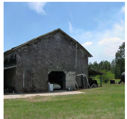
Existing large rustic barn
