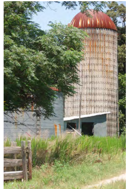
Silo at Long Valley Farm
