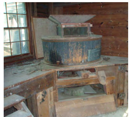
Interior of Mill House
