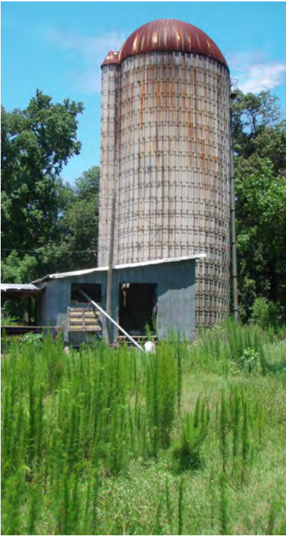
Silo and Silo Shed
