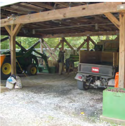
Typical park maintenance facility
