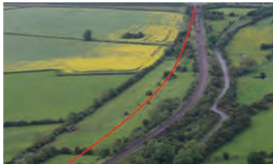
Figure 10.1 Line speed improvement project new alignment at Market Harborough
