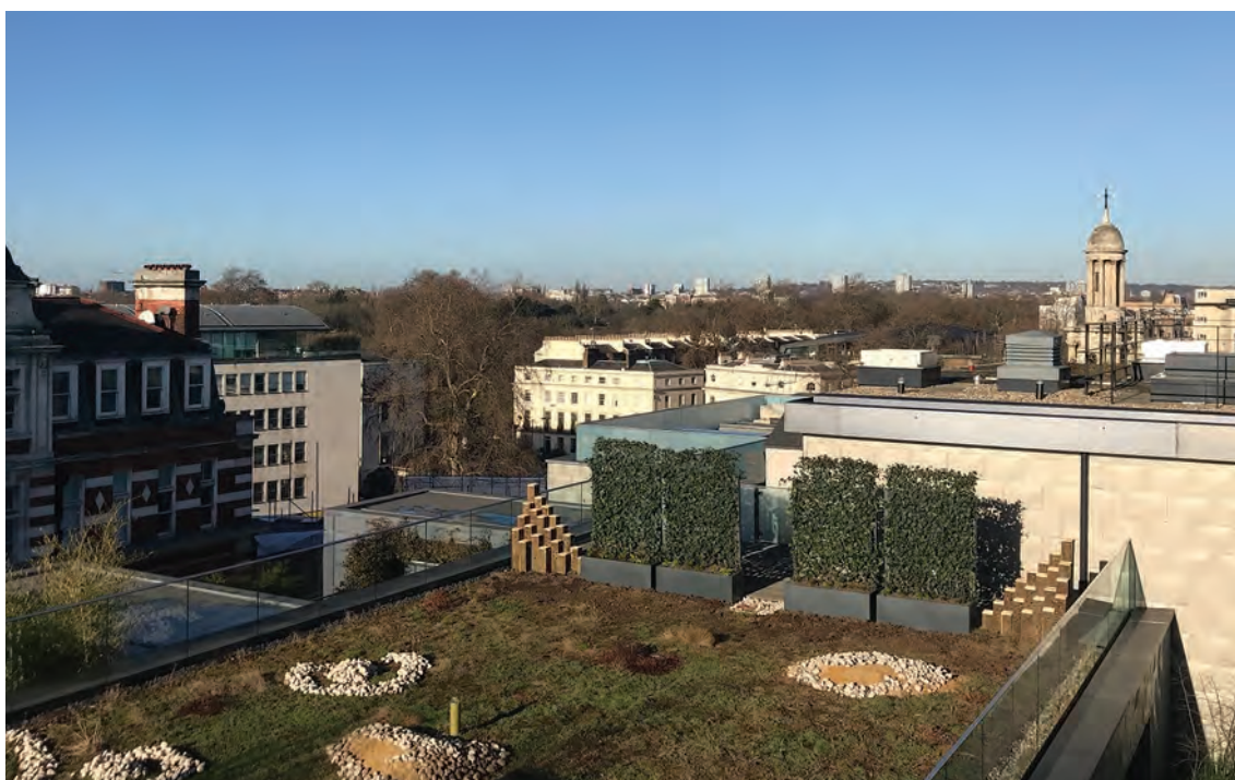
Figure 27.1 Augmented living roof at 50 Bolsover Street
