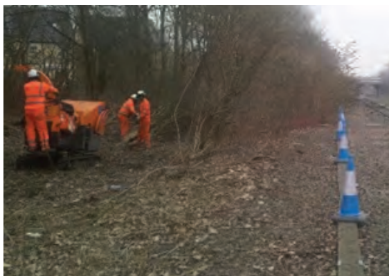
Figure 9.1 Vegetation clearance for Carillion's Midland Mainline programme projects
