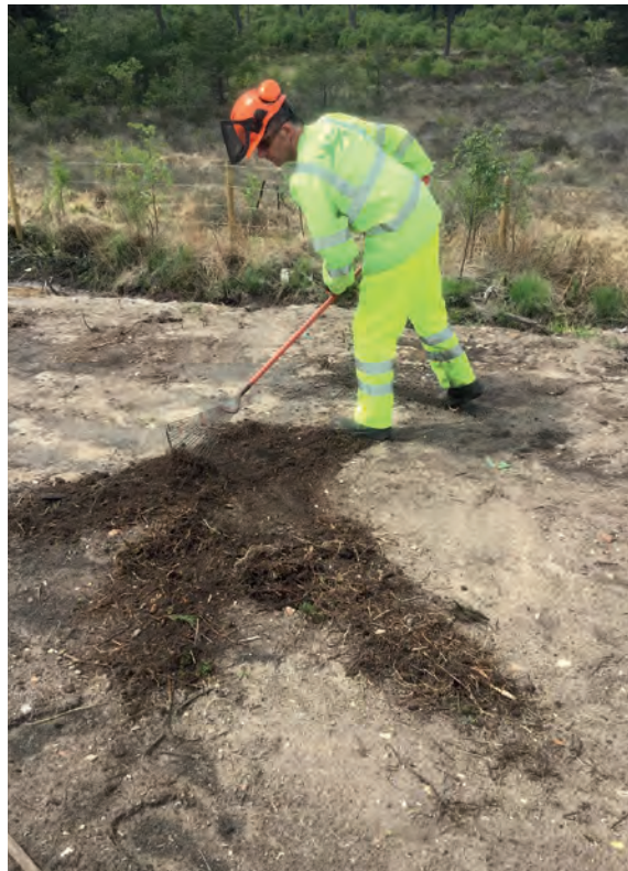
Figure 4.3 Spreading heather brash on the new road verge to encourage creation of heathland vegetation
