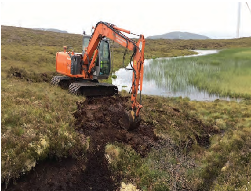
Figure 23.1 Restoration works (before)
