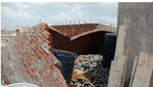
Figure 2: Under Construction Vault Roof
