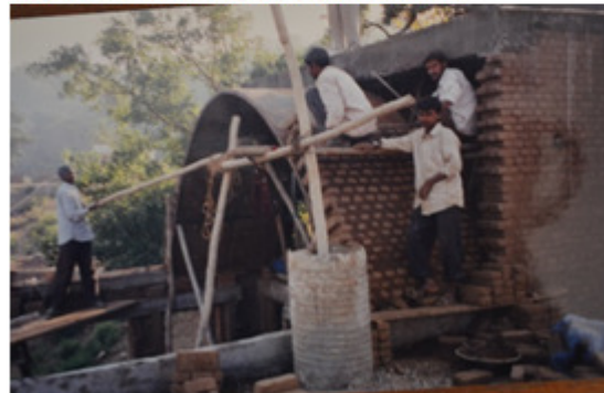
Fig. 9. Vaulted roof construction.
