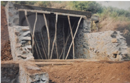
Figure 6: Plinth Construction for House
