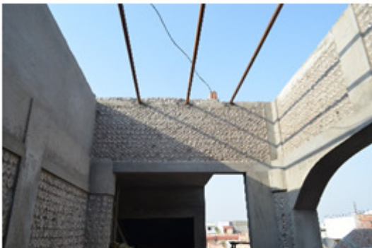
Figure 1: PET Bottle in Walls and Columns
