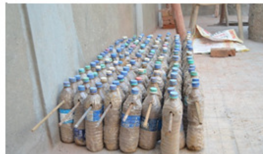
Figure 3 PET Bottles ready for Installation
