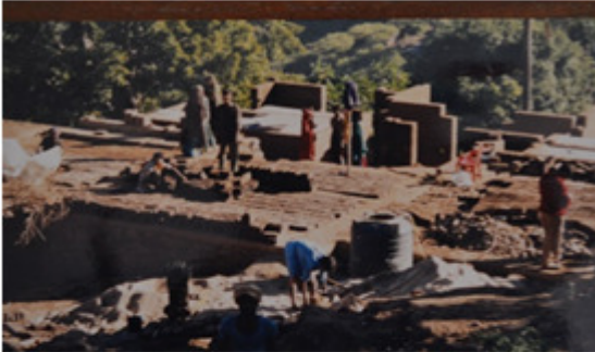
Figure 10: On Site Drying of Mud Blocks
