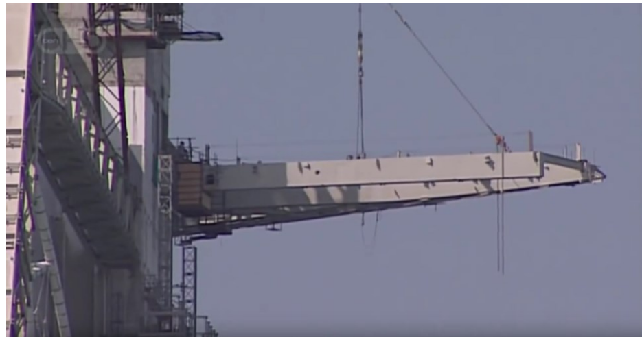
Sky view restaurant: survives wind 160 km/hour aluminium, glass, steel frame Box girders 27 m projected each side, 200m above sea
