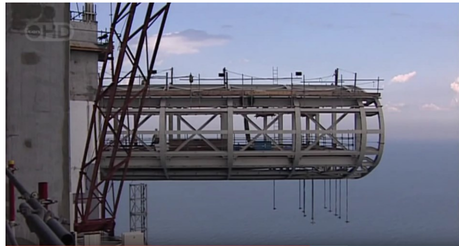
Sky view restaurant: survives wind 160 km/hour aluminium, glass, steel frame Box girders 27 m projected each side, 200m above sea
