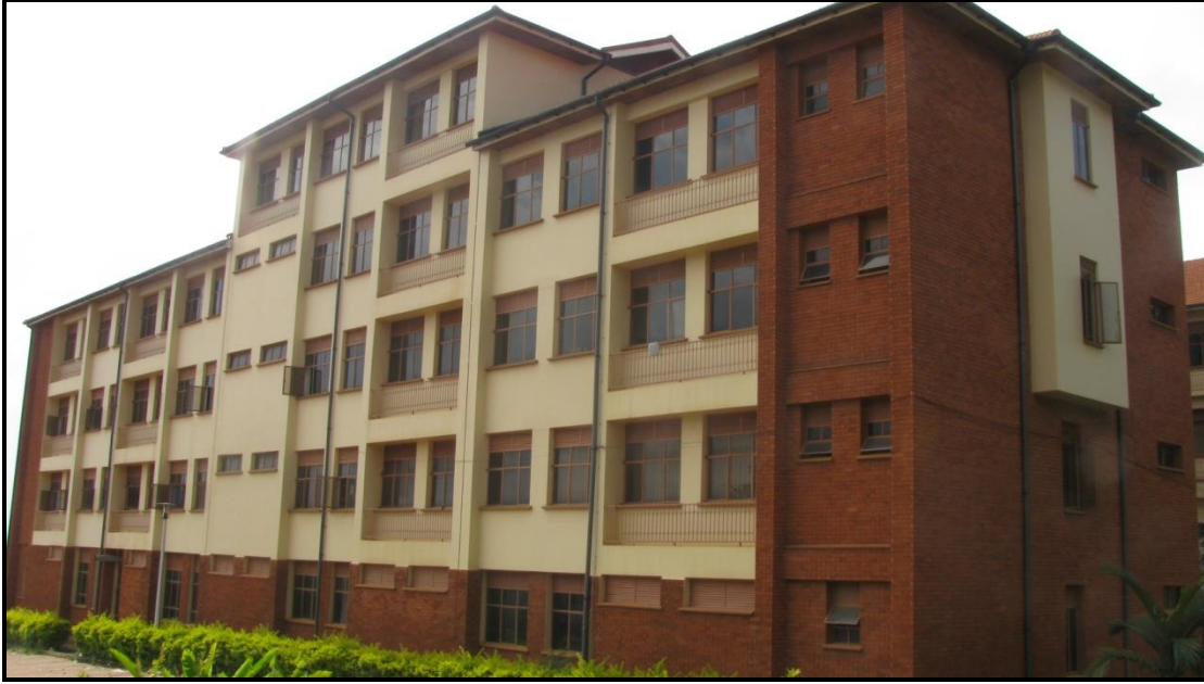
Figure 3. 1: Building main facade and surroundings
