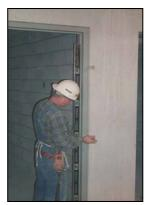
Figure 5: Inserting Wooden Shims
