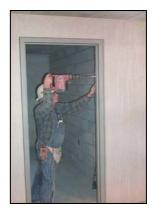
Figure 6: Drilling for Anchor Bolts
