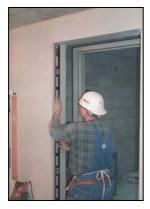
Figure 4: Drawing a Plumb Line
